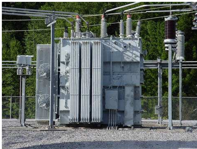
Figure 9.20: Substation transformer.
